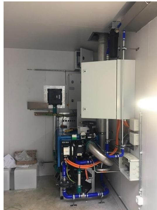
The Ballard MD-30 fuel cell has a rated net power of 30kW in dimensions (l x w x h) of 900 x 480 x 375 mm weighing 125 kg. Full specs are here. The fuel cells that will be used in the full-scale drive train are the HD100 with a 100 kW rated net power, with dimensions of 1200 x 869 x 506, weighing 285 kg. Full specifications are here.
